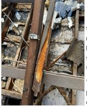
the roof to make sure the roof was stable and would last for many years. The new timbers are a different colour to the existing timbers.
